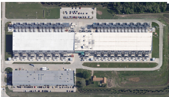
A Google data center in Council Bluff, Iowa
